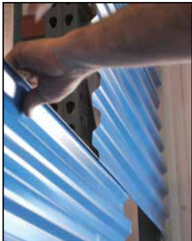
Hang panels on hooks, no fasteners yet
