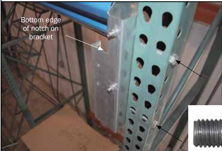
Bottom edge of guide flare aligns with bottom of notch in door mount
