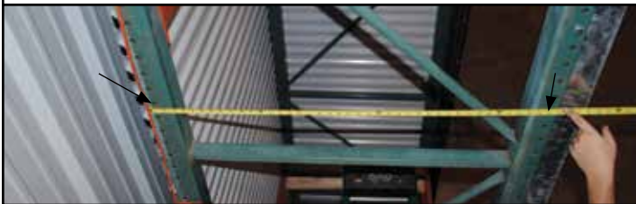
Measure to use the existing pallet rack holes to install tube
